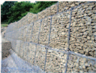
gabion filtration wall
